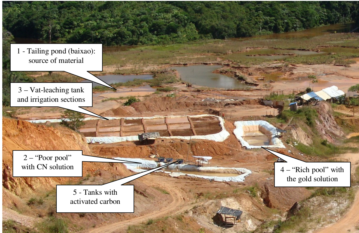
Figure 4 – General view of the vat-leaching process
